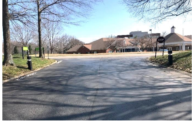
Eastbound Comdata North Entrance at Winners Circle
