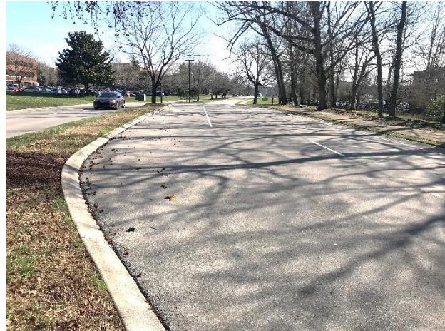
Eastbound Maryland Way at Continental Place
