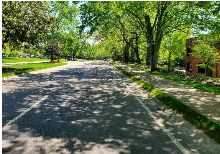
Eastbound Maryland Way approximately 315 feet west of the Comdata access
