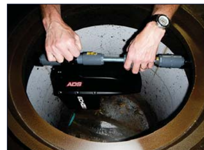
ECHO with installation bar mounted on manhole frame
