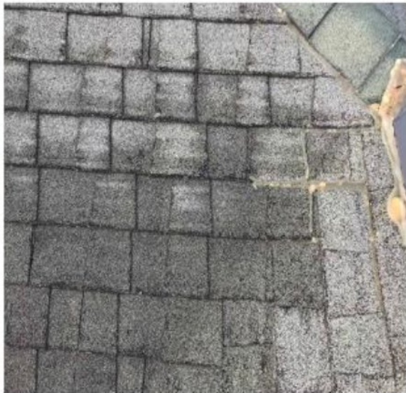
Shingle deteriorated
