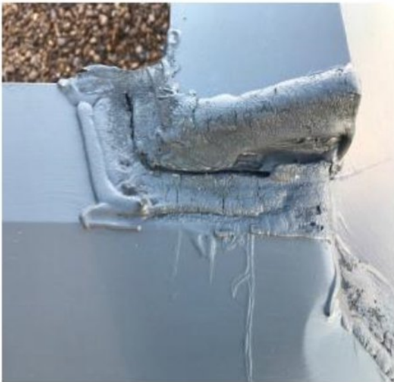
Open at top of coping of shingles
