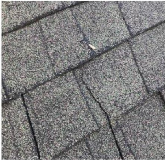
More shingles cracked in the area of Leak
