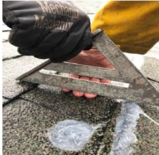
A hump was in shingles probably caused by buckled sheathing. Water ponding under this condition can enter roof at shingle joint below it.
