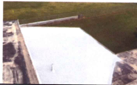
Above, is the first area where the restoration system was applied. It took everything adjusted and set up the first time, so it was the only area completed. We expect nearly 15,000 square feet of application on a good day.
