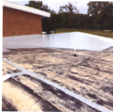
Above, is the first area where the restoration system was applied. It took everything adjusted and set up the first time, so it was the only area completed. We expect nearly 15,000 square feet of application on a good day.
