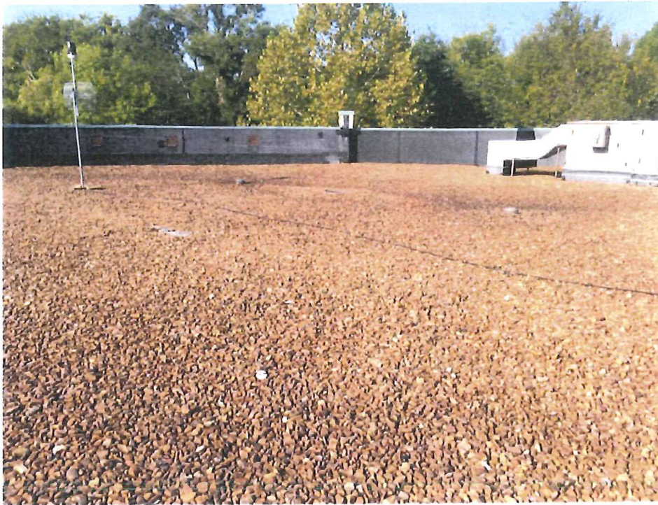
This is a photo of the roof field.
