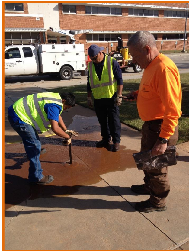
Figure 7. Visual Observations – Our personnel will make visual observations of water distribution system issues/damages as we proceed through the process of localization and pinpointing of leaks.
