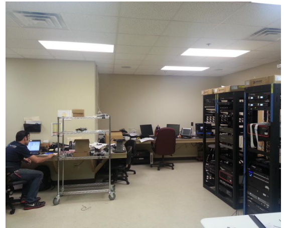
M3 staging facilities are used for system pre-fabrication and testing
